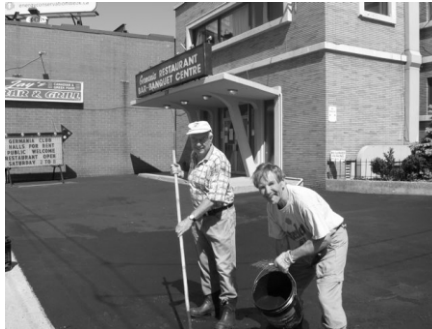
The next two Days Arthur and Eckhard applied Driveway Sealer on the asphalt.
